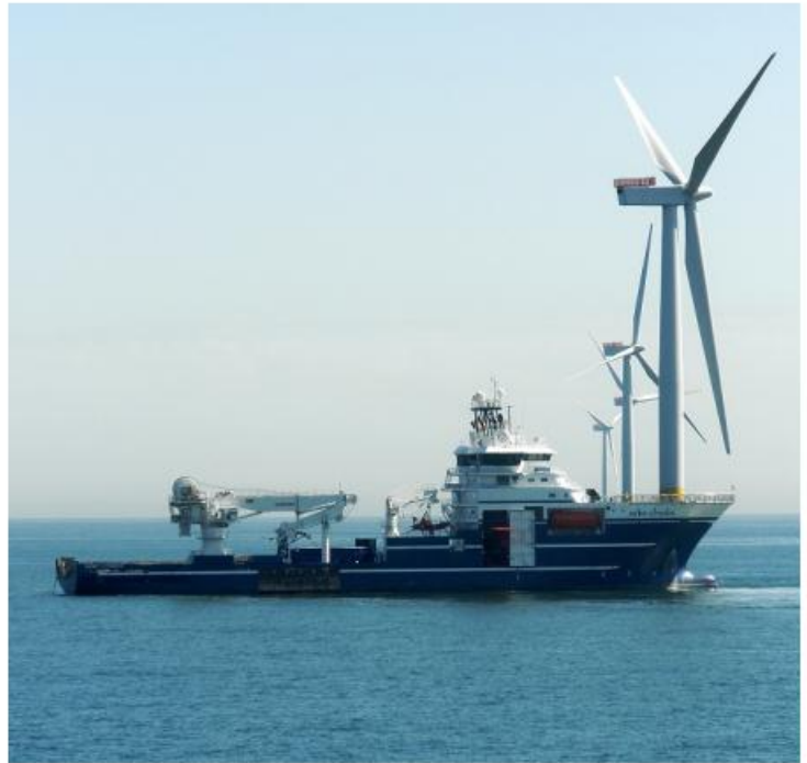
Deep Cygnus performing trenching and cable burial operations at the Greater Gabbard Offshore Wind Farm in the North Sea
