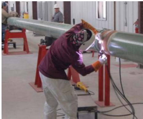
Helix Danny pipe-in-pipe welding
