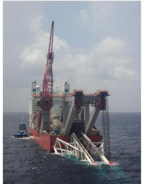
Caesar installing EOG Toucan pipeline offshore Trinidad
