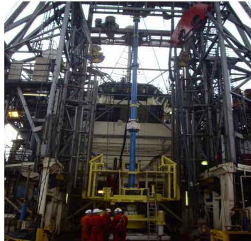
7 1/16" SIL in the Seawell Derrick
