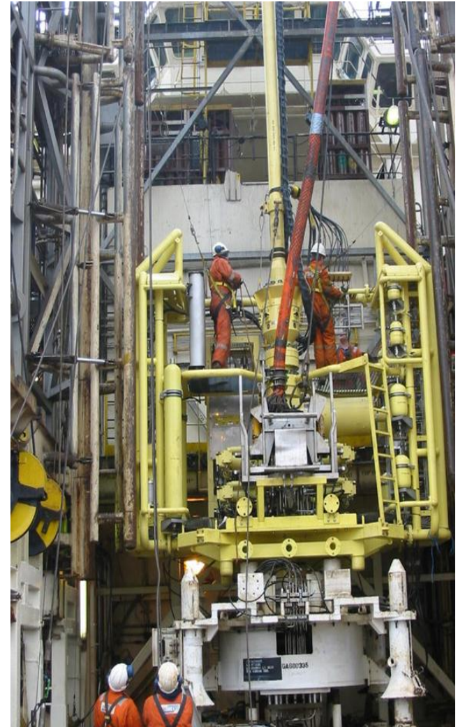
5 1/8" SIL in the Seawell Derrick
