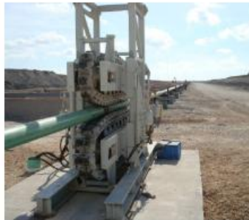
Automated pipe tension system
