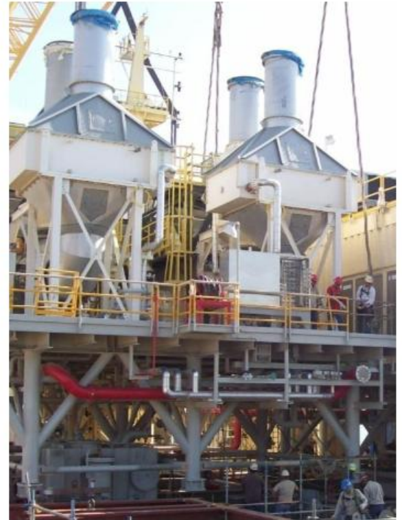
HPI production module installation
