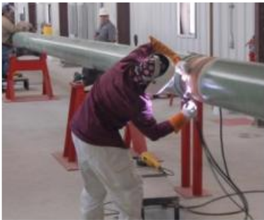
Helix Danny pipe welding
