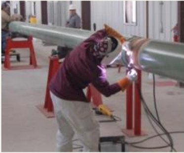
Helix Danny pipe welding
