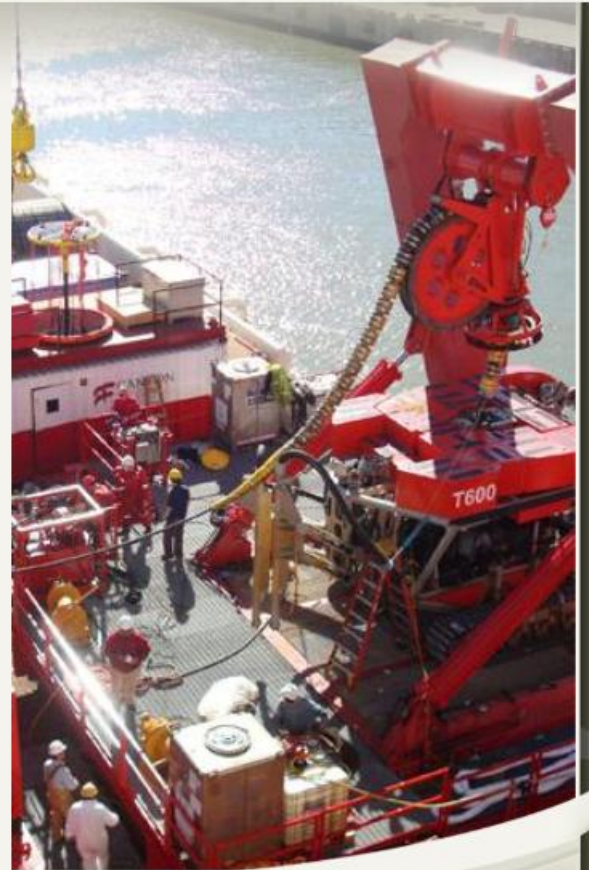
Canyon Trencher ROV mobilization
