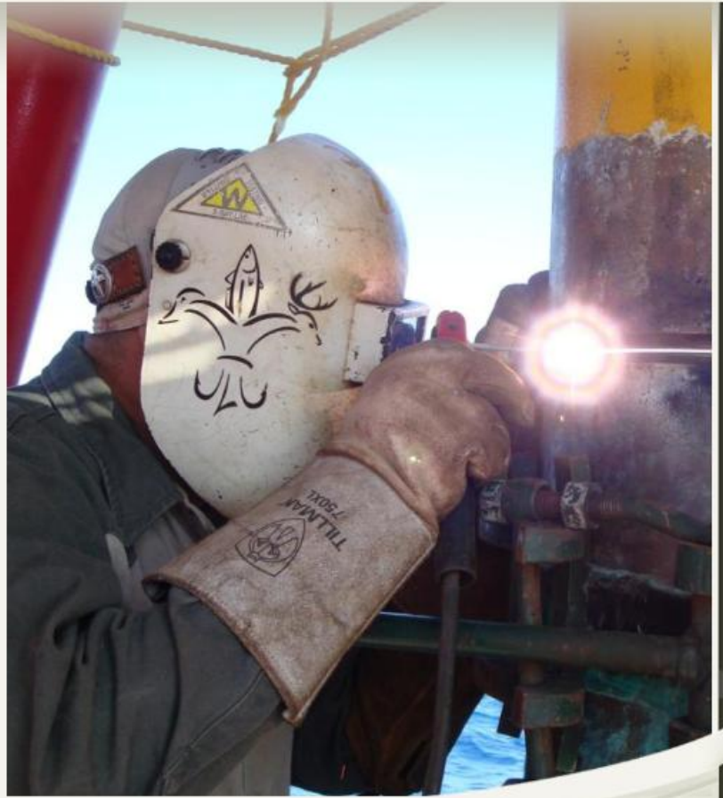
Pipeline to PLET welding for ENI Longhorn
