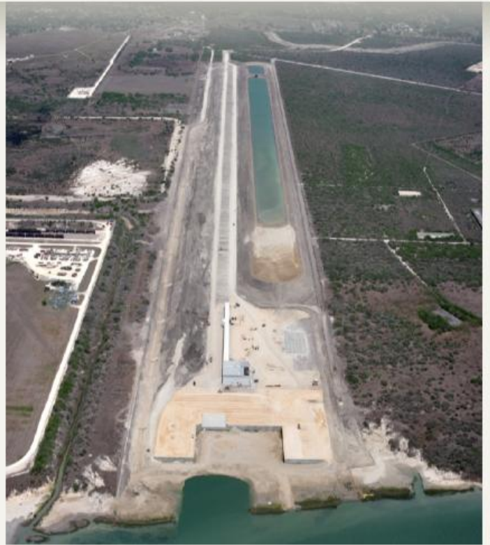
Aerial view of Ingleside Spoolbase, with slip dredging project underway
