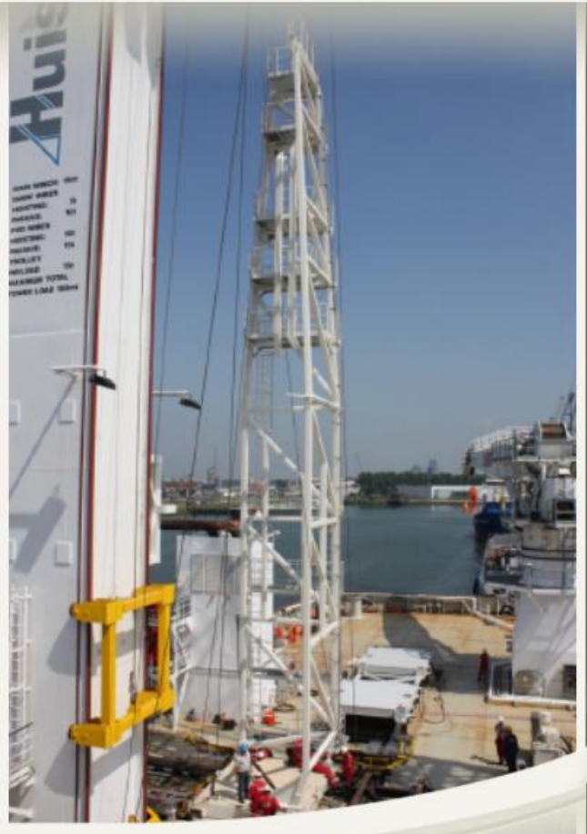
Subsea Intervention Lubricator access tower installed on Well Enhancer deck
