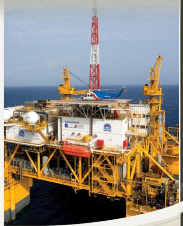
Independence Hub production platform
