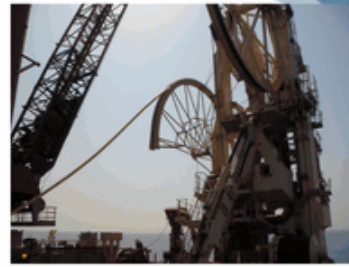
Express working on Reliance KGD6 project Offshore India
