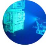
Intervention Riser Systems (Gulf of Mexico)
