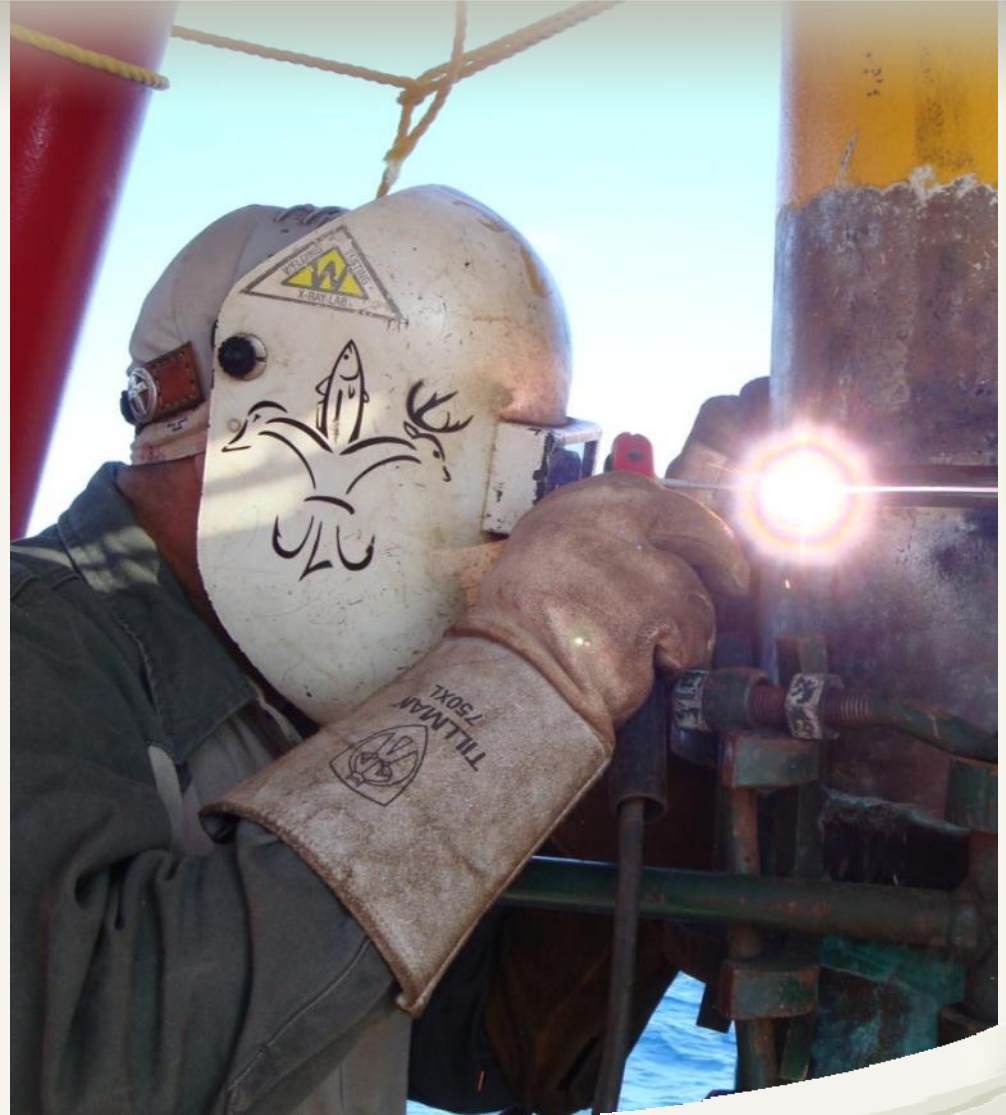
Pipeline to PLET welding for ENI Longhorn
