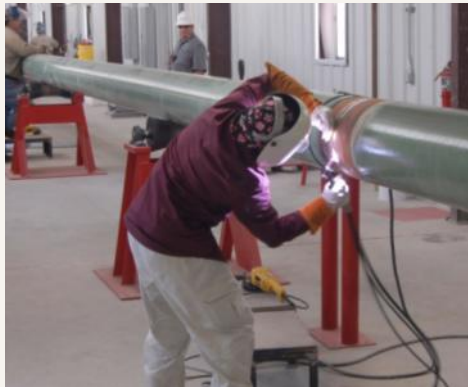
Helix Danny pipe welding
