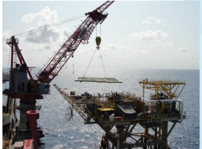
Helideck installation utilizing the Caesar
