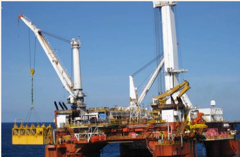
Q4000 installing ENI Longhorn manifold
