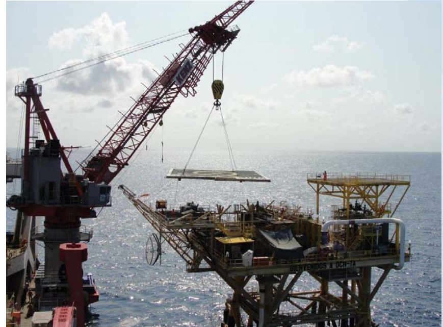
Helideck installation utilizing the Caesar
