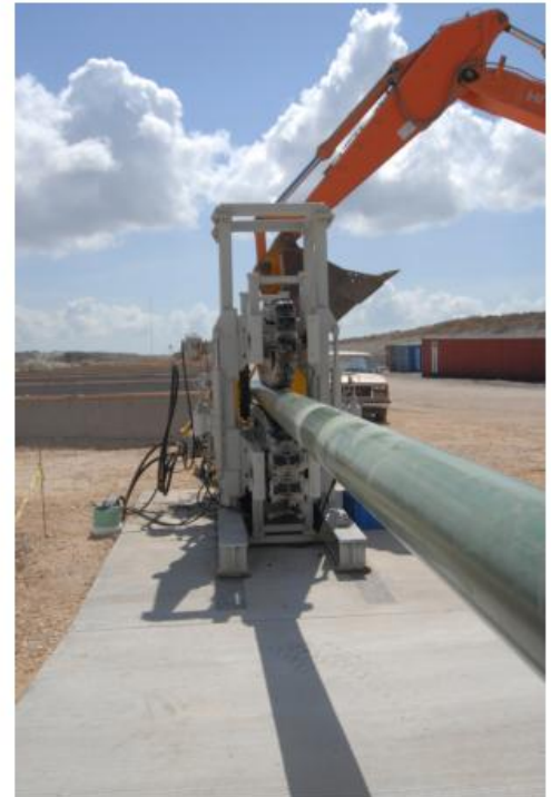
Welding and spooling pipe at Ingleside Spoolbase
