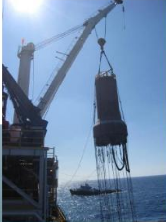
DTS Buoy being installed by Q4000
