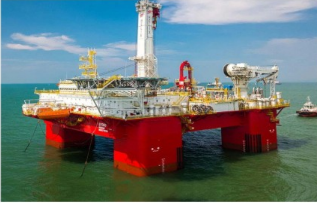
Q7000 – Under Completion
