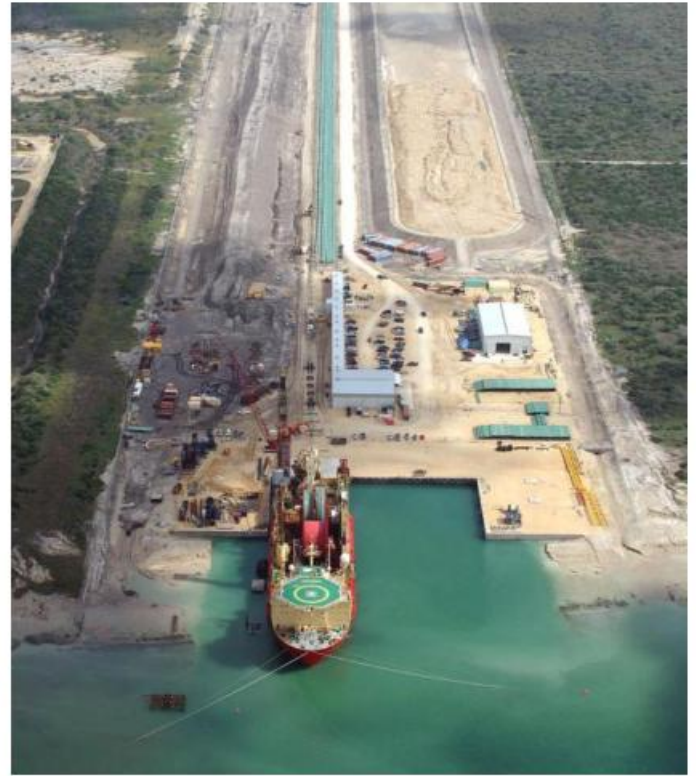
Aerial view of Ingleside Shore Base
