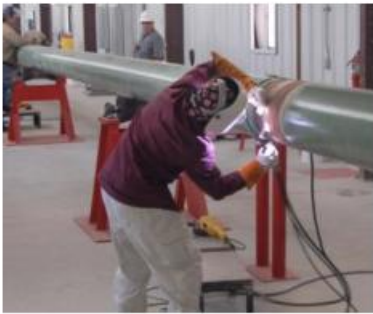
Helix Danny pipe-in-pipe welding
