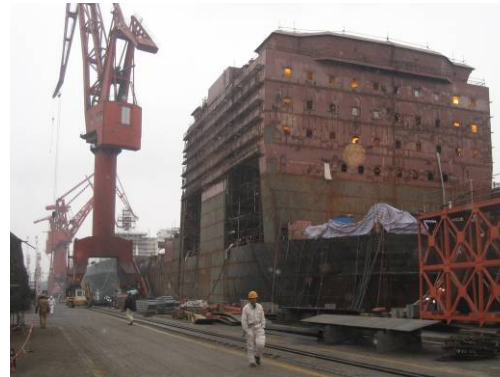
Conversion of Caesar underway in China
