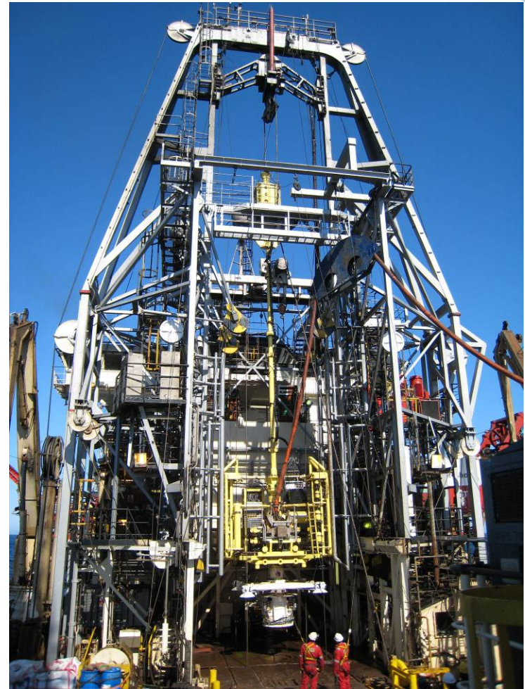
Subsea Intervention Lubricator stack-up on Seawell
