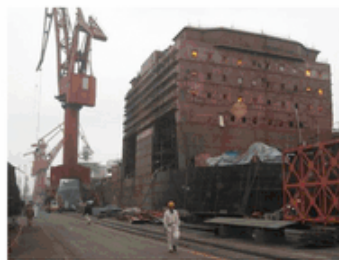
Conversion of Caesar underway in China
