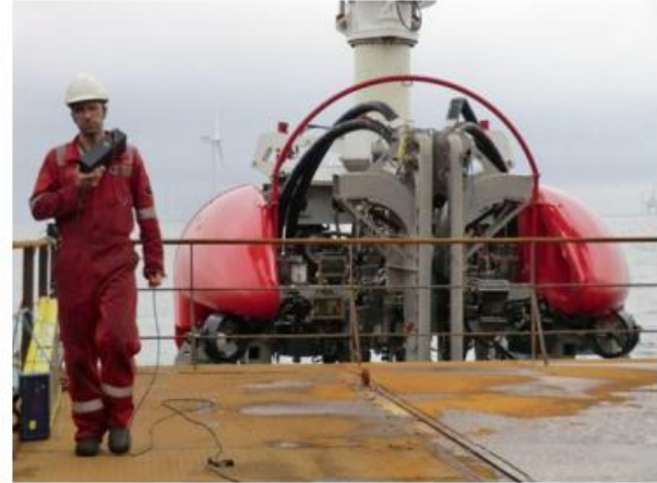
T1200 trencher being deployed
