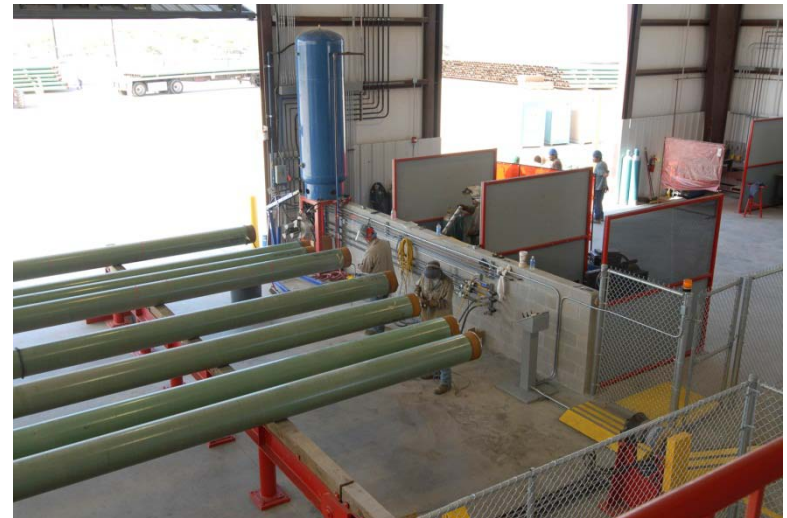
Ingleside Spoolbase Facilities
