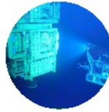
Intervention Riser Systems (Gulf of Mexico)
