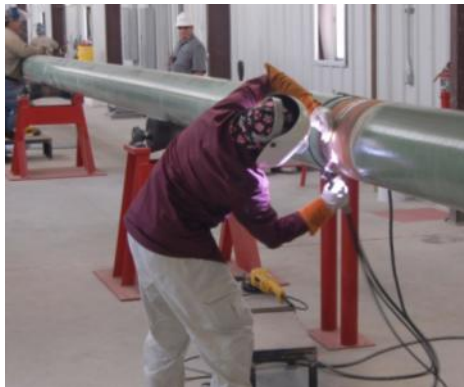
Helix Danny pipe-in-pipe welding
