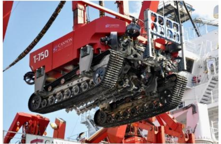
T750 trencher being launched from the deck of the Island Pioneer
