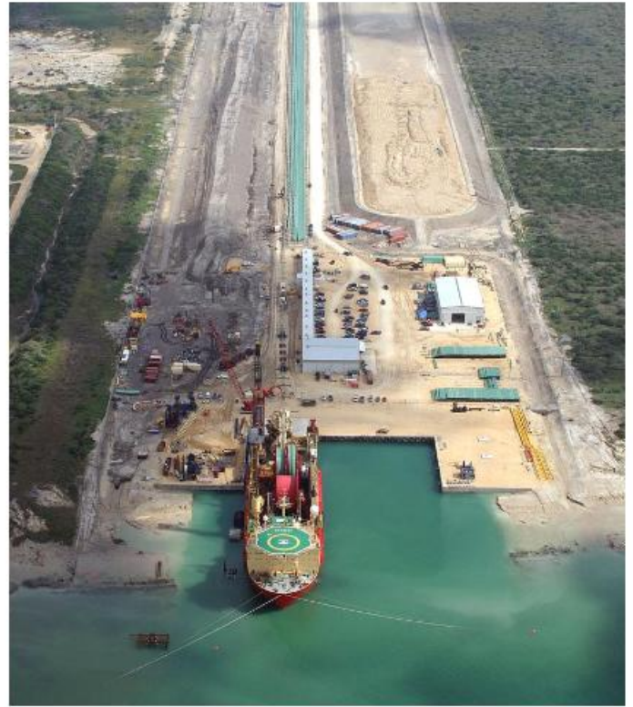
Aerial view of Ingleside Shore Base
