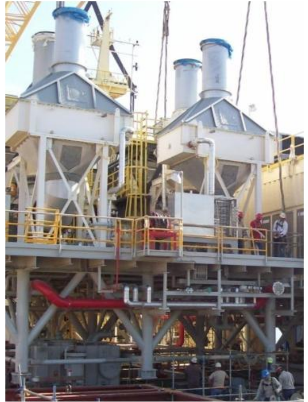
HPI production module installation
