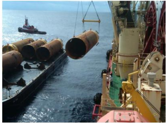
Express installing suction piles in the Walker Ridge block of the Gulf of Mexico
