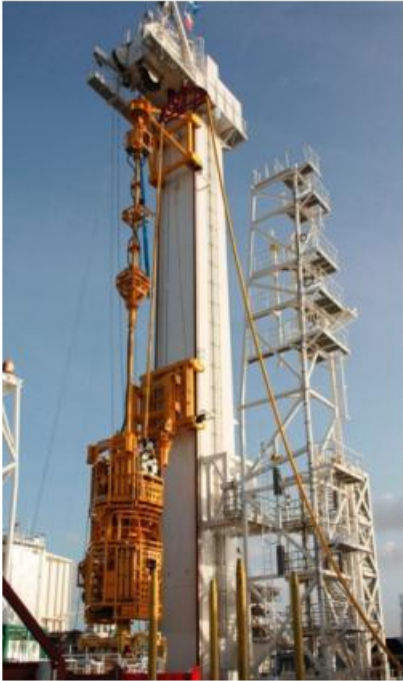
7 3/8" SIL in the Well Enhancer Tower
