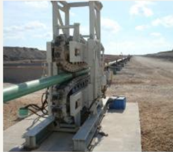
Automated pipe tension system
