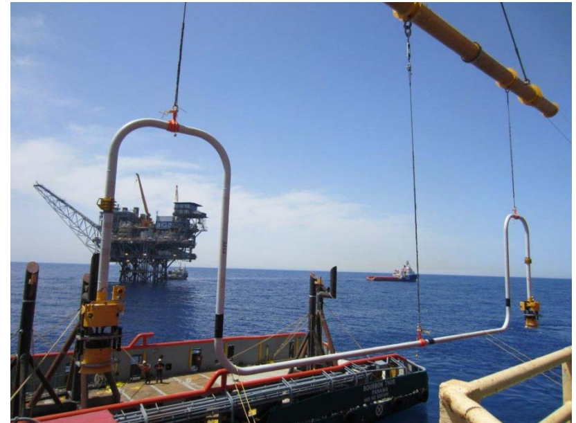
Express installing a jumper in Noble Energy's Noa field off the Israel coast.
