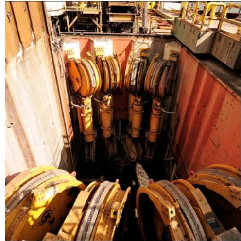
Q4000 moonpool during drydock in Brownsville, Texas
