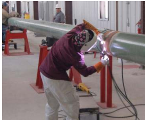
Helix Danny pipe-in-pipe welding
