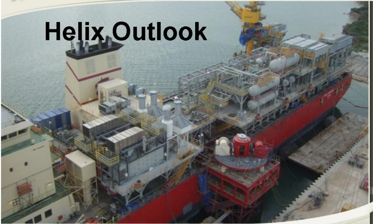
Helix Producer I topside module installation progress at Kiewit Offshore Services fabrication yard
