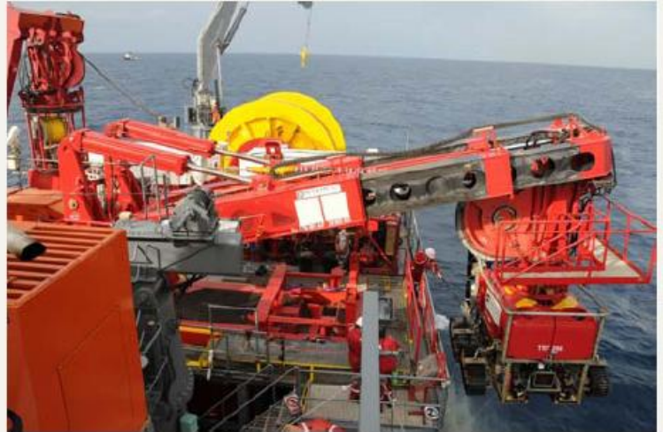
Cable trencher T200 being launched from the Seacor Canyon offshore Indonesia
