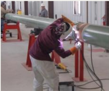
Helix Danny pipe welding
