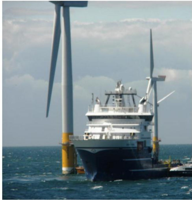
Robotics business unit at work in UK windfarm
