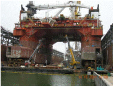
Q4000 enters Dry-dock in Galveston for marine and drilling upgrades
