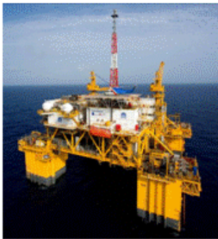
First production at Independence Hub occurred in July
