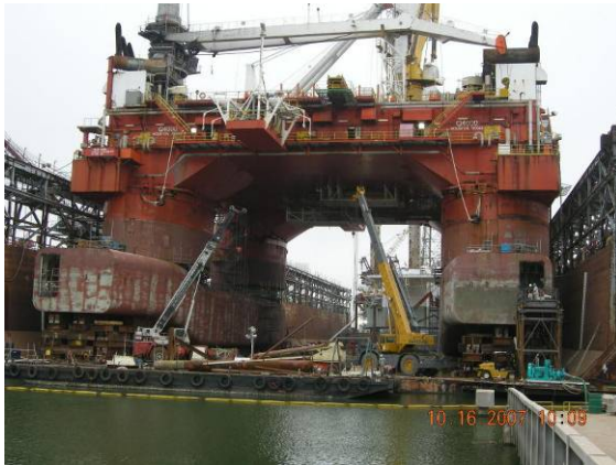
Q4000 enters Dry-dock in Galveston for marine and drilling upgrades
