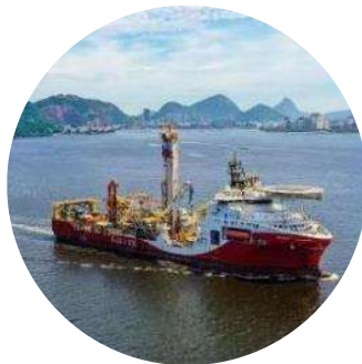
Siem Helix 1 & Siem Helix 2 (Brazil) DP3 well intervention vessels contracted through at least 2027 (SH1) and 2028 (SH2)
