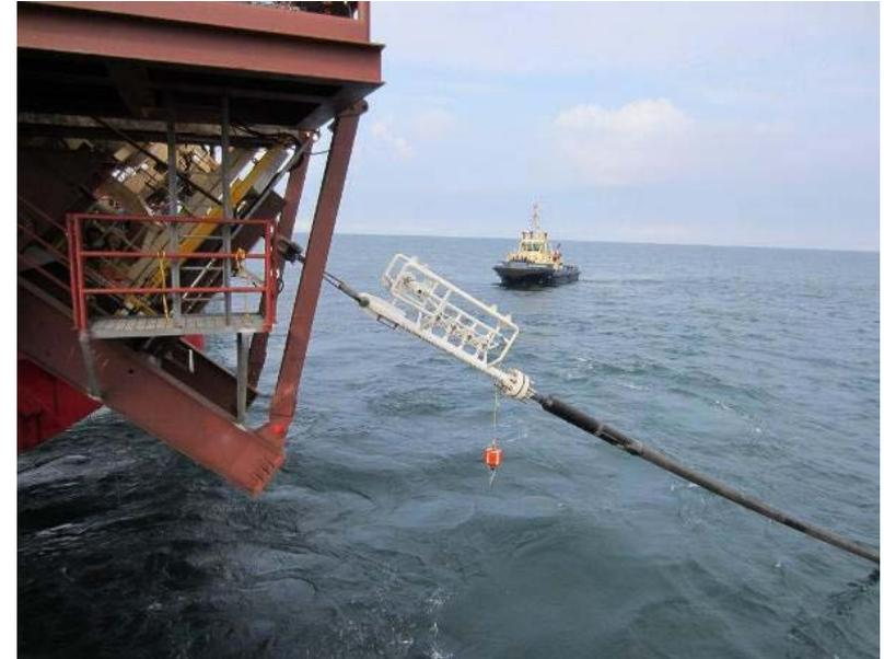
*Express lowering a pipeline pullhead as part of a North Sea installation operation.*
