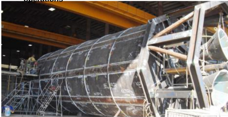
New buoy for HPI under construction
