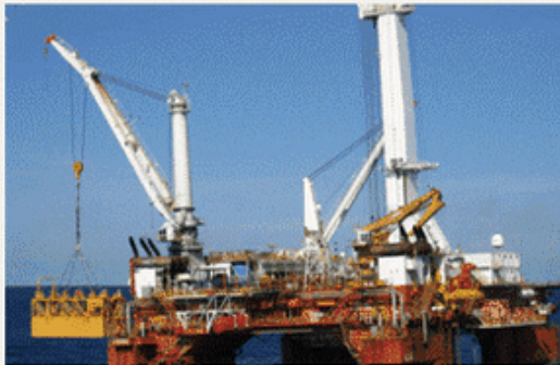
Q4000 installing ENI Longhorn manifold
