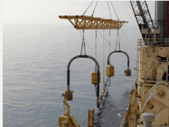
24-inch deepwater jumper being installed by Express on Reliance KGD6 Project offshore India
